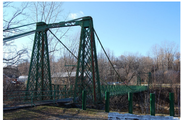
Pedestrian Suspension Bridge- Keeseville
