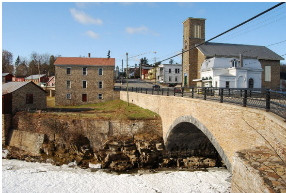
Keystone Arch Bridge- Keeseville
